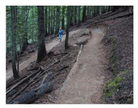
There were also exposed tree roots at the upper end of the trail segment, with measured dropoffs of up to 19". For this project, we focused on short trail realignments in some areas in order to reduce the grade. At the top of the climb, a realignment wasn't possible, so we instead installed crib steps. We built the crib steps to standards established by the US Forest Service as appropriate for multi-use trails, including both equestrian and mountain bike travel.
