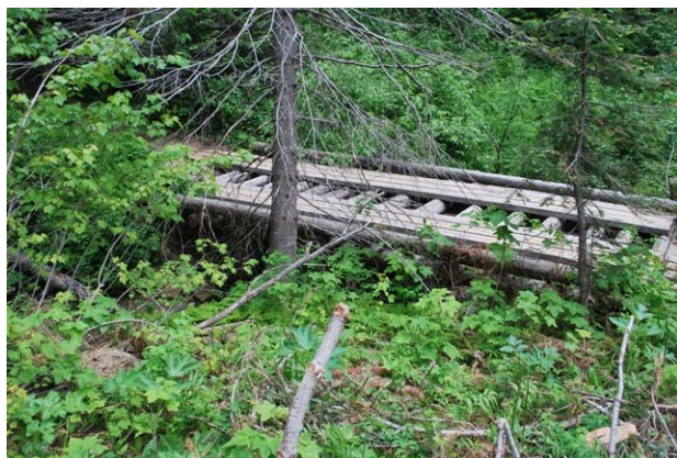
2009 view of bridge remaining over Deadman Creek.
