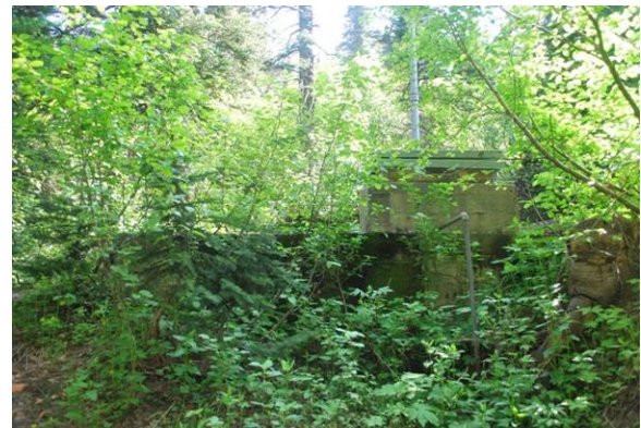
2009 view of reservoir from below.
