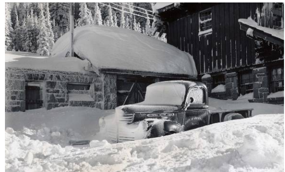
Garage at east side of Lodge. WSPRC Photo 78.2003.1.P319A.U1 (January 3, 1944).
