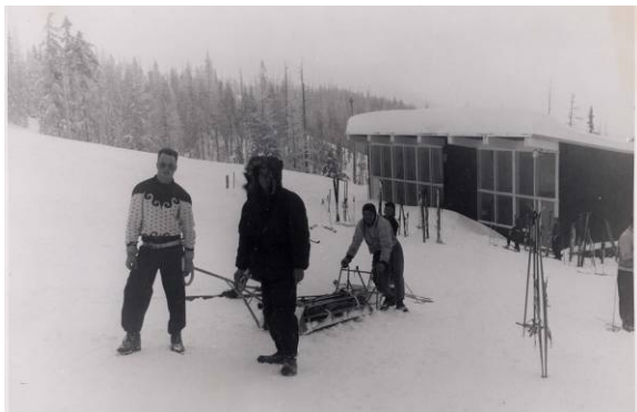
Historic view of Lodge 1, prior to additions.
