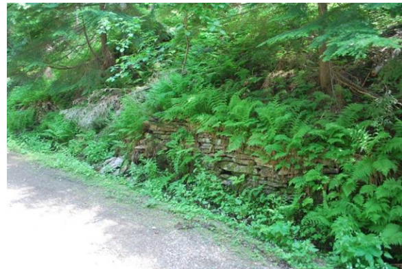
2009 view of revetment shown at left.
