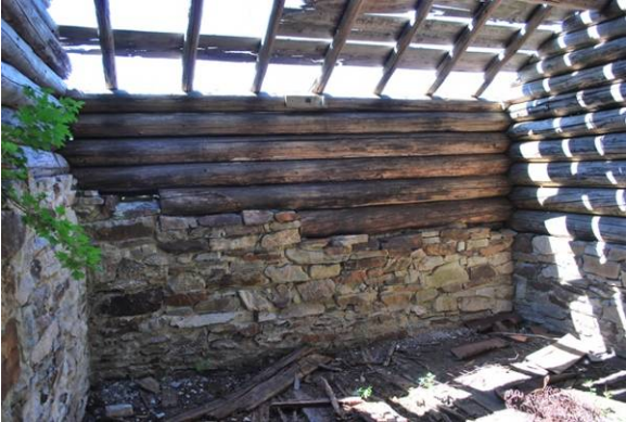
2008 view of Woodshed interior.
