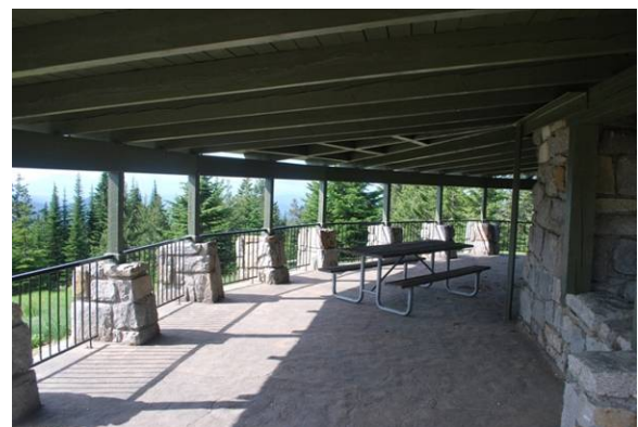
2009 view of interior to west.
