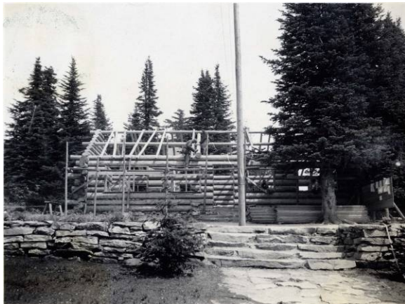
Under construction, 1934. WSPRC Photo SP10-60.
