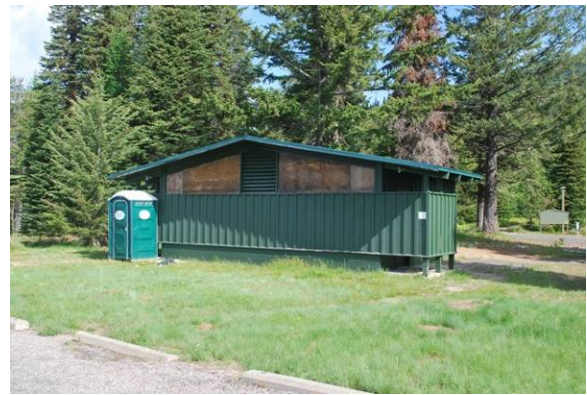
2009 view to north.
