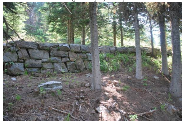
2009 view of stone wall.
