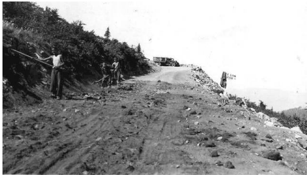
Switchback near Cook's Cabin area, July 1935 Photo SP10-184
