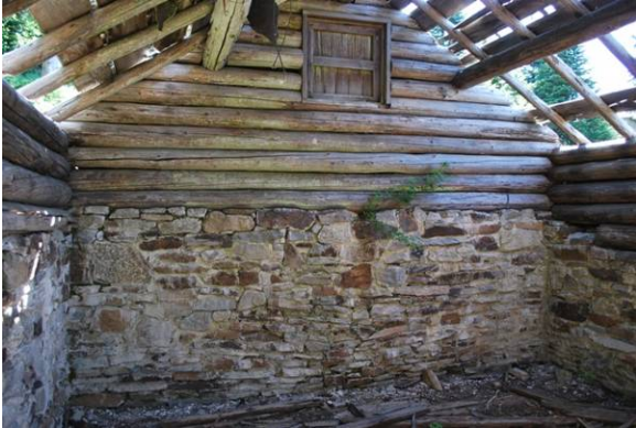
2008 view of Woodshed interior.
