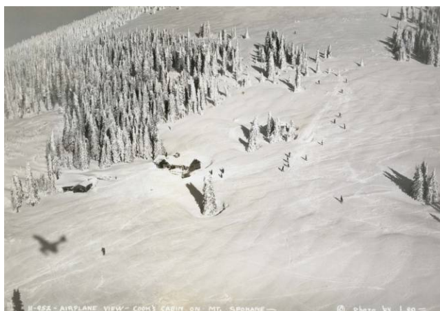
Aerial view of Cook's Cabin (far left) and Caretaker's House (left center). Latrine in cluster of trees at center. WSPRC Photo 78.2003.1.P975A.K4
