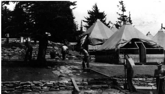
Camp construction, July 1934. Photo SP10-143.
