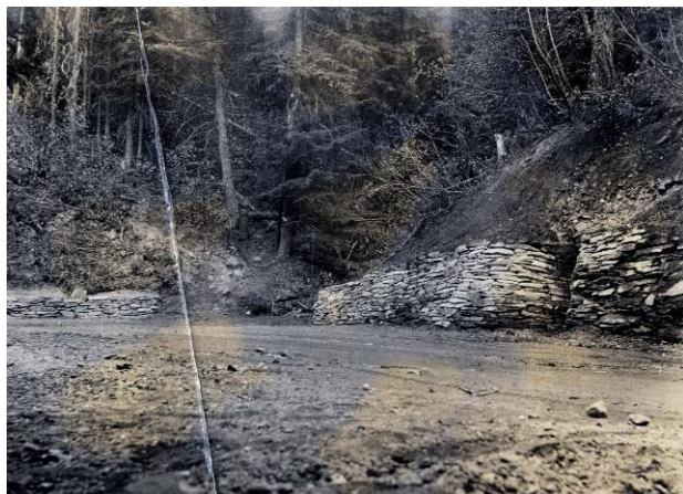
Stone revetment along Kit Carson Road, October 1934. Photo SP10-81.
