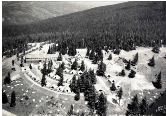
Aerial view of Camp Cook. WSPRC Photo 78.2003.1.P1062D.V4.
