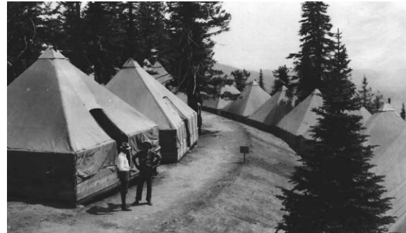
Completed camp segment, July 1934. Photo SP10-7.
