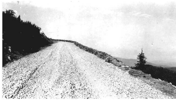
Project complete, October 1935. Note rock wall to right. Photo SP10-193
