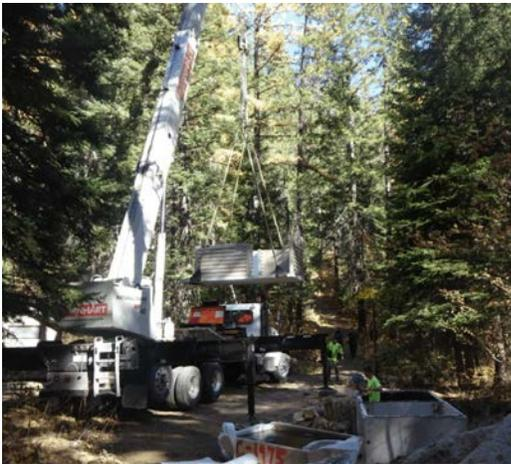
It was delivered on two very long flat bed trailers and a special crane was needed to fit the pieces together. The second trailer was too long to make it around two tight corners, so it was chained to the big excavator to prevent it from sliding completely into the creek. In the end, it was a successful installation that has already proven its value.
