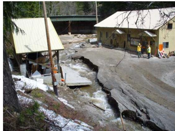
Quick work by Park staff last May 18 prevented a flood in the headquarters building, but didn't prevent about 1000' of state highway from washing away. Water was flowing around a blocked culvert under the sand shed at an estimated 38,000 gpm. The road was rebuilt quickly, but a larger culvert will need to be placed under the road this summer when the first mile of Park road will also be rebuilt. The Park road is expected to be closed again all summer.
